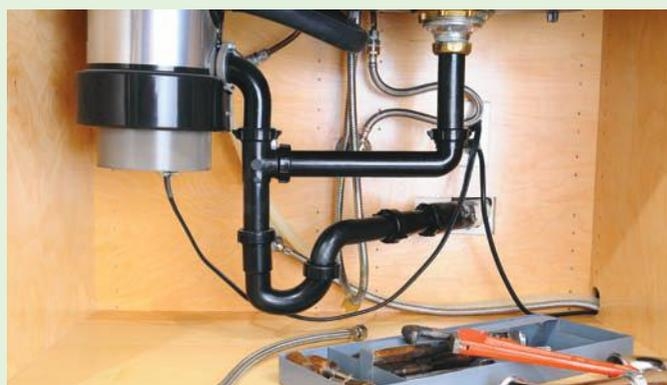
Figure 14.17 These pipes are made from PVC.
