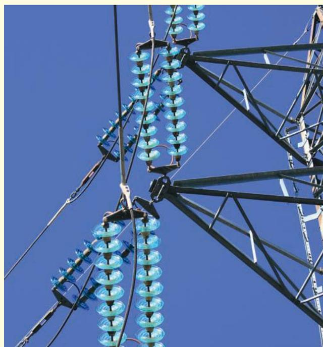
**Figure 3.39** Ceramic discs prevent short-circuits in the national grid.
