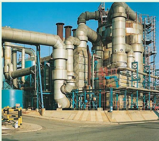
Figure 12.7 A Contact process plant used for making sulfuric acid.
